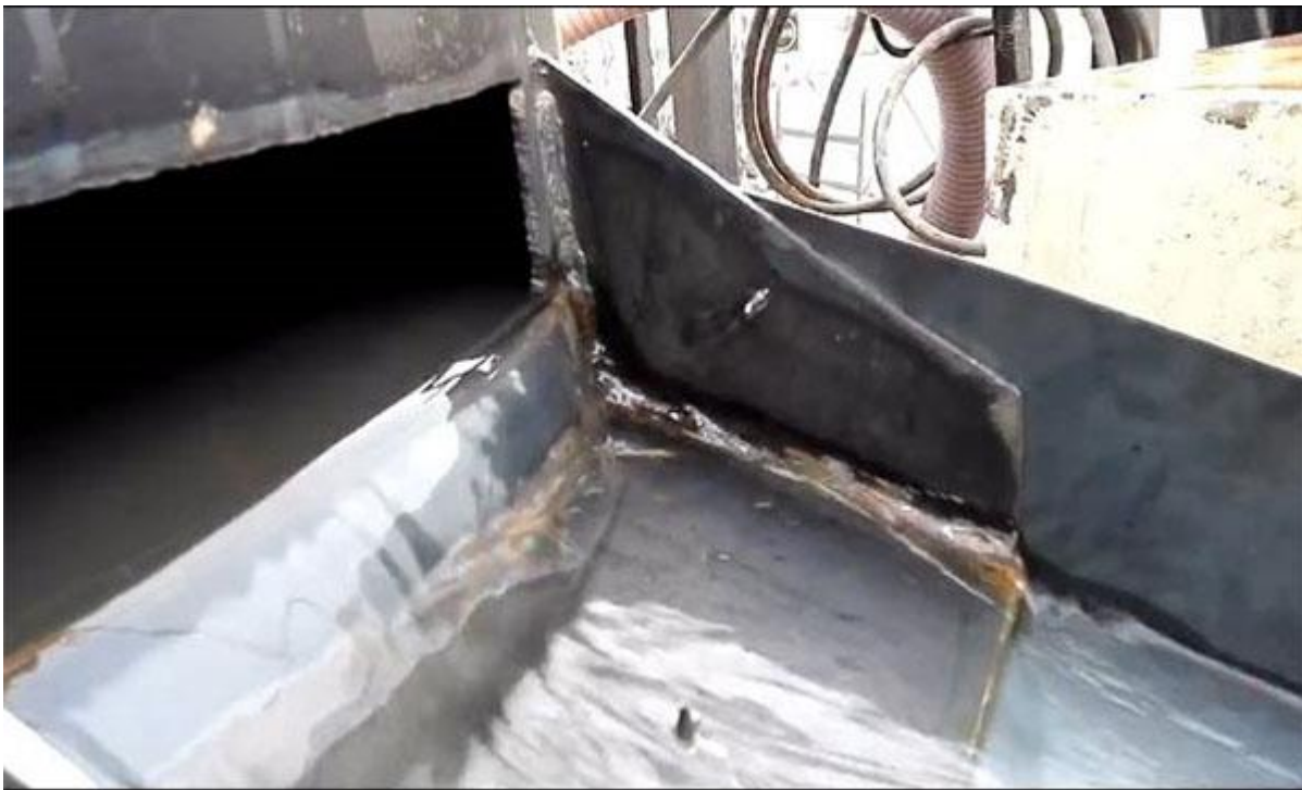
c. Solid waste dry discharge dry discharge and dry heap treatment of solid waste in tail water
